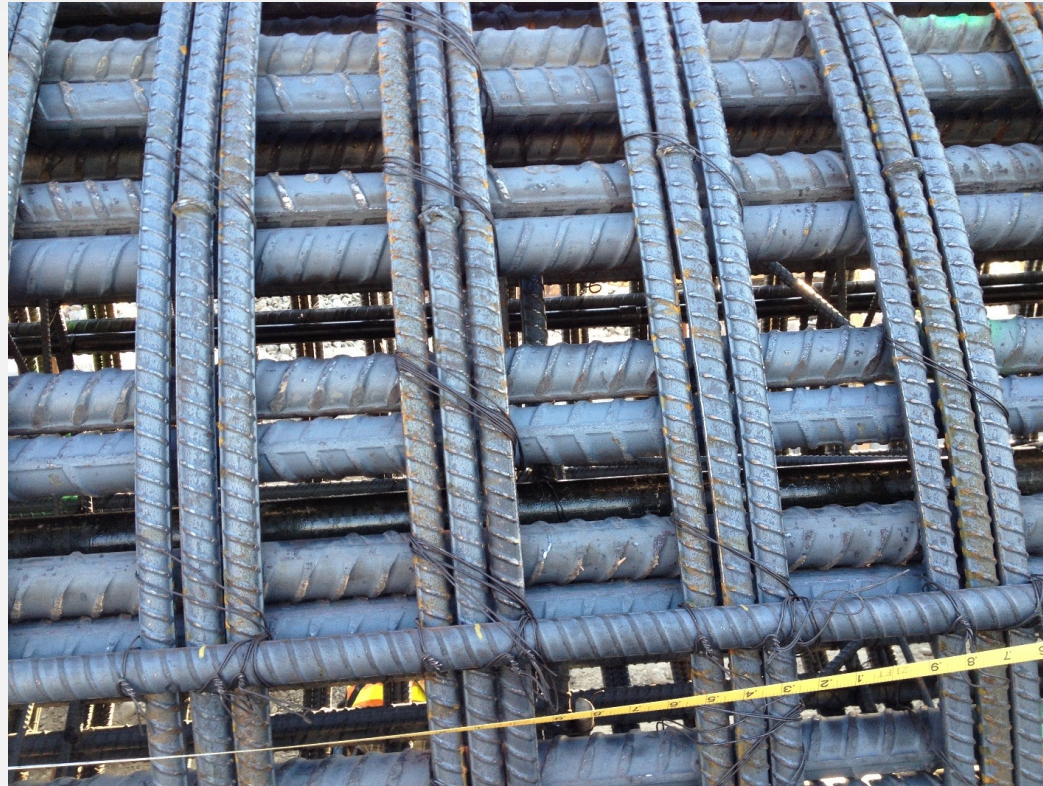
BUNDLED BARS AND HOOPS
