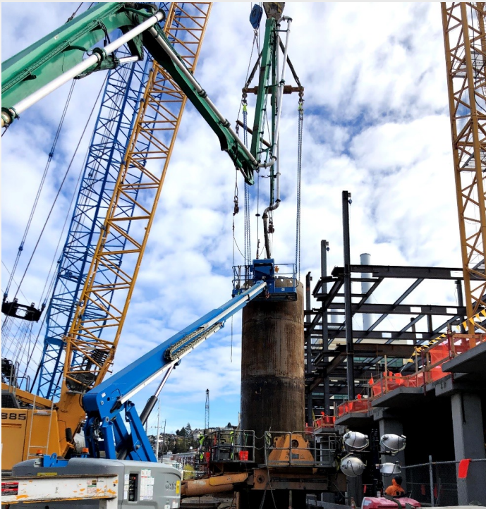
PUMP DIRECTLY INTO TREMIE
