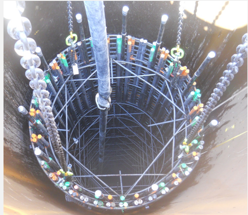
HOLD CAGE WITH CRANE
