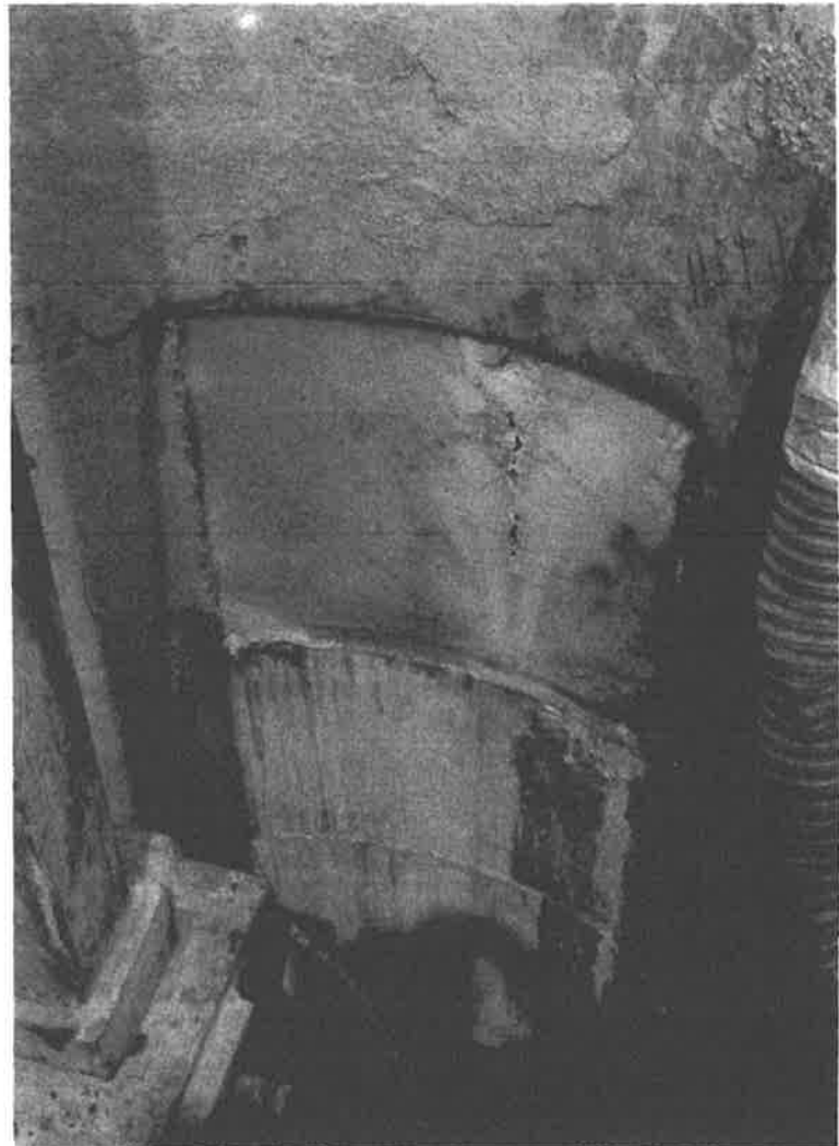
Photos 17 and 18 Removal of the access windows and revealing of the cement grout which was placed outside the access casing to a depth of 60 feet to minimize groundwater infiltration during construction and observation.
