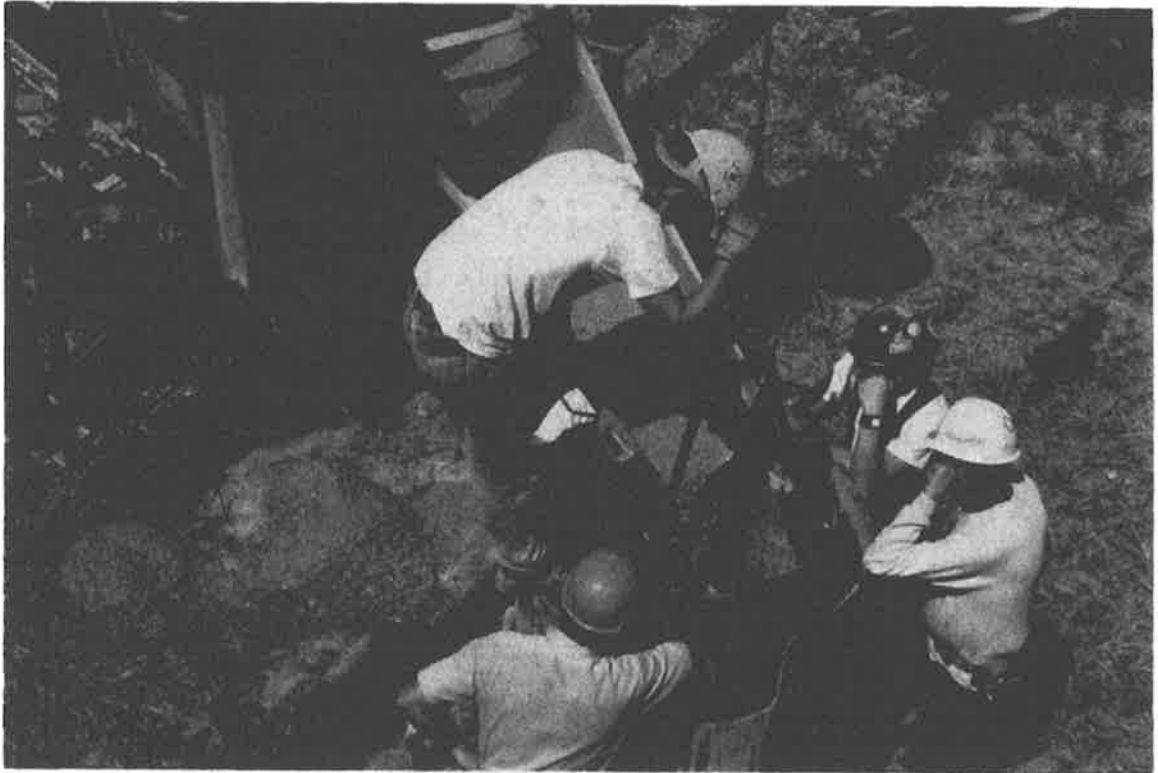
Photos 11 & 12 Concrete placed by the tremie method into the East caisson at a depth of 53 to 65 feet using Mix #4 with a 7 inch slump. A 12 inch diameter rigid steel tremie and hopper were used. The bottom of the tremie pipe remained embedded within the fluid concrete at the bottom of the lift during the pour.
